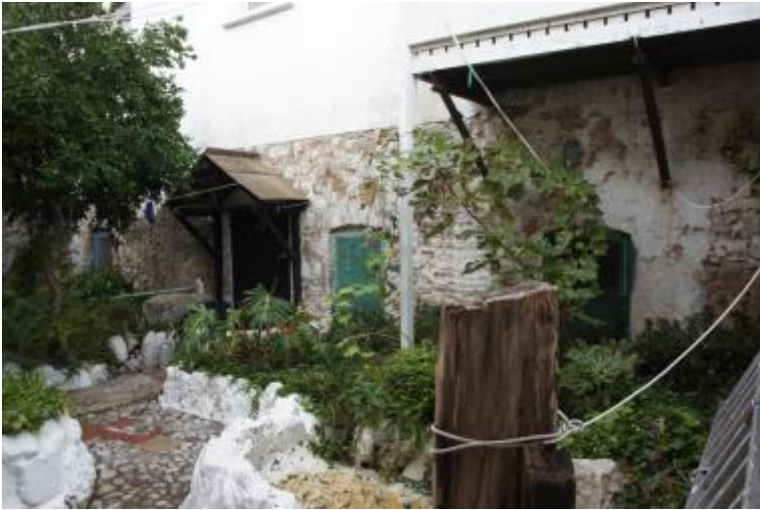
Toc H Hostel abutting the walls
